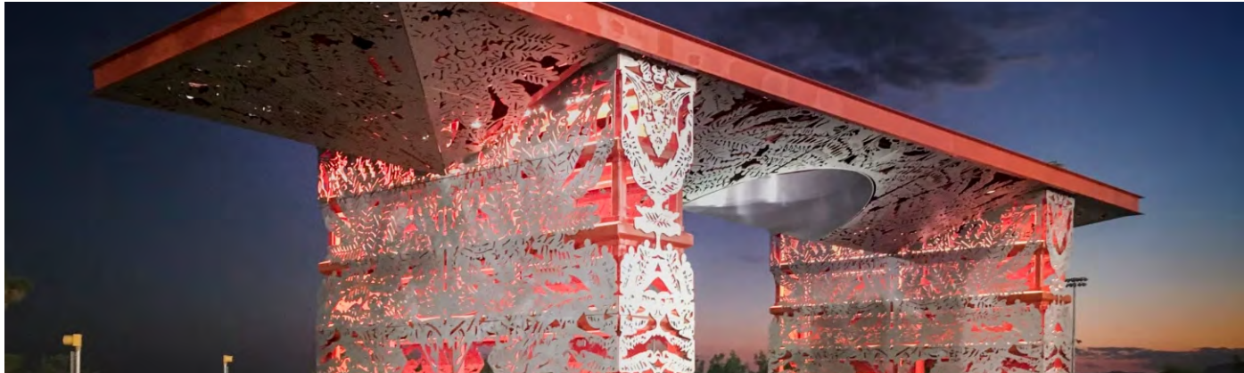
Figure-13 : Sun Pavilion At Night | Photo @ A. Zahner Company
