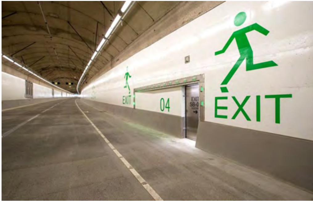
Figure-81: The Highway 99 tunnel north portal, near Harrison Street, heads south under downtown Seattle to the stadium district. Signage shows drivers where the nearest escape exit is in case of an emergency. (Mike Siegel / The Seattle Times)
